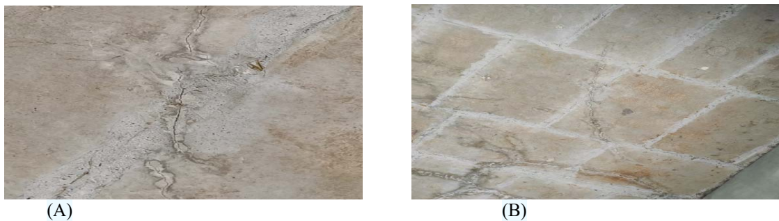
Figure 1: A. and B. cracks pattern at the bottom of the slab
