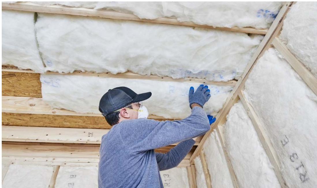
Figure 2 : Installation of fibreglass insulation in the walls and ceilings [9]
