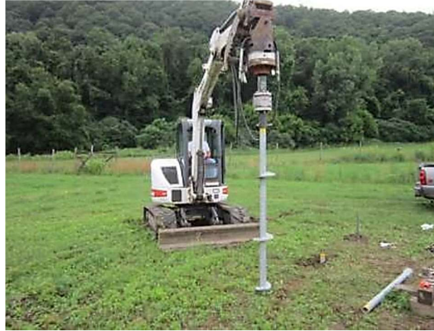
Figure 2: Drilling of Helical Pile [16].
