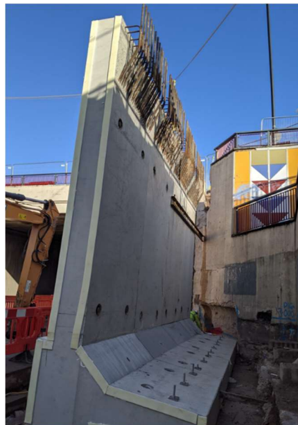
Figure 10 – Installation of OSM abutment panels, back view of the panels [Photo courtesy of Tarmac]
