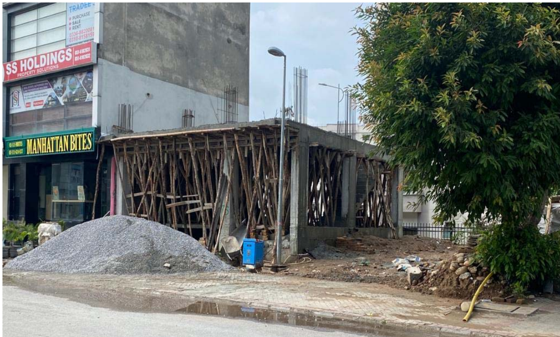
Figure 2: Conventional method of commercial building construction in Pakistan.
